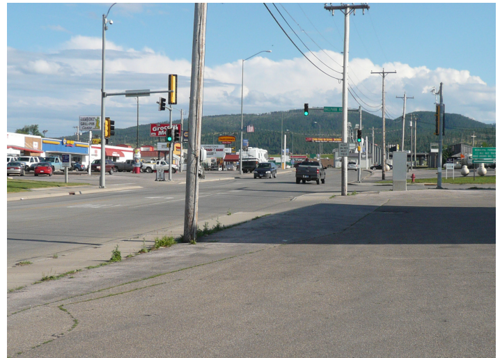
The south segment of Junction Avenue. A combination of hard surfacing, conflicting driveway accesses, and a continuous center left-turn lane creates both safety and aesthetic challenges along a main gateway route to Sturgis.
